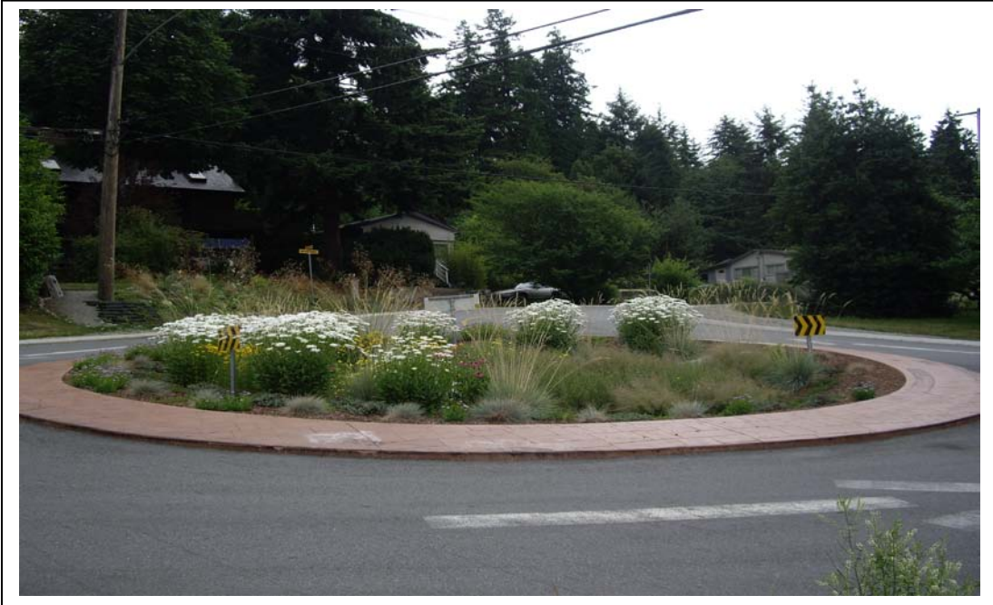
Stormwater catchment traffic calming circle. Photo from 2009.
