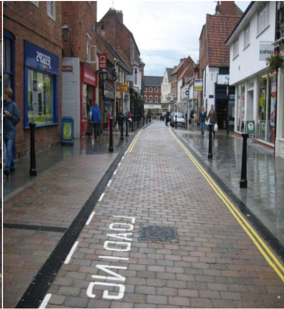
11. Middlegate following completion of work. Late 2007
