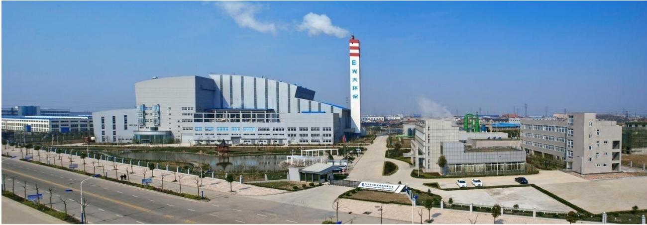
A refuse incineration power plant capable of processing 1,200 tons waste per day was constructed.
