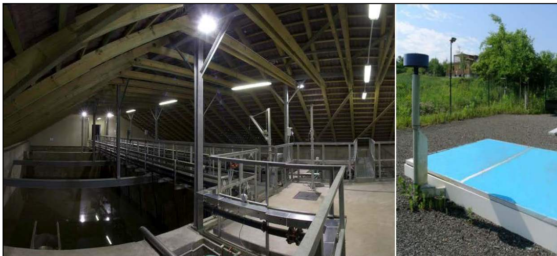
Sewage treatment plant in Kladno-Vrapice and small sewage treatment plant for Čabárna village – June 2012
