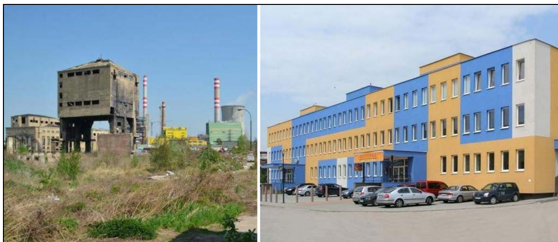
Old part of Enterprise Zone Kladno-East – May 2012
