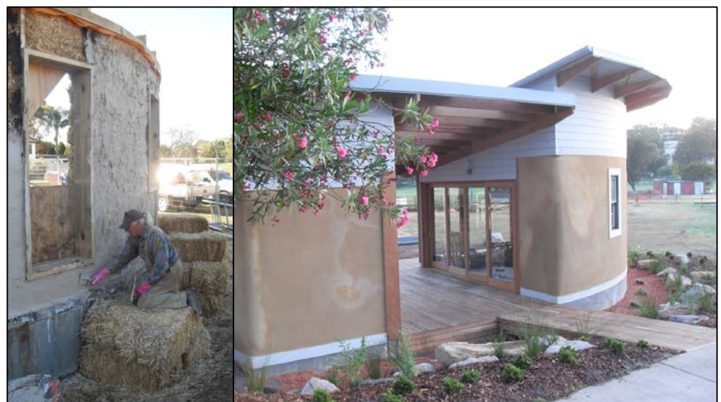
Figure 15: The Carss Park Eco-shed - built from straw bales with recycled tyres as foundation instead of a full concrete foundation. Rainwater tanks were also installed. (February 2009)
