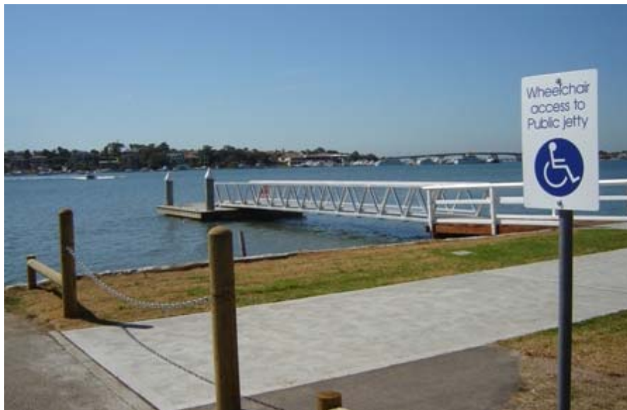
Figure 19: The Disable Access Jetty at Dover Park Boat Ramps, allowing sailors with disabilities to sail on Kogarah Bay (February 2012)
