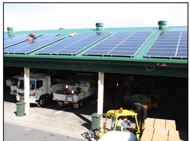
Figure 11: Kogarah City Council's Solar Depot Project where 216 solar modules were installed with a capacity of 37.8 kilowatt. The solar panels reduce approximately 40% of the Depot's annual energy use. (2010)
