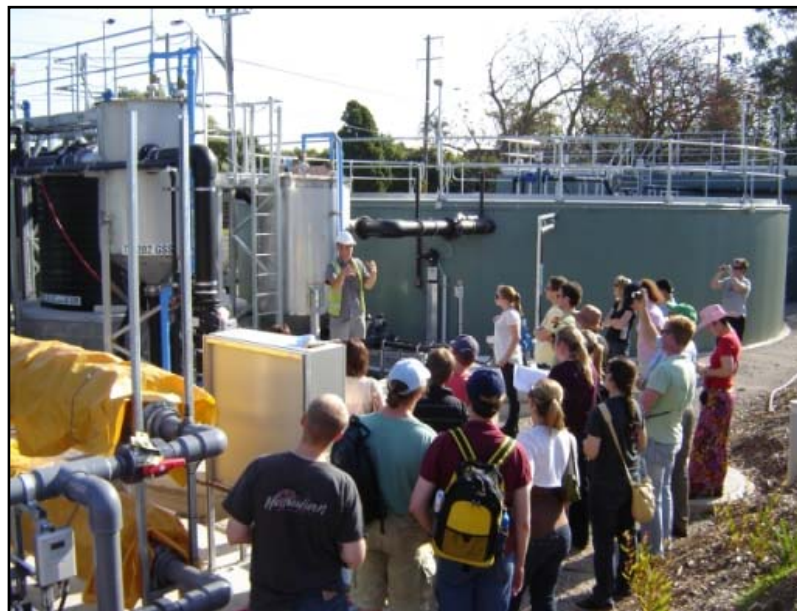
Figure 9: A tour of the Beverley Park Sewer Mining Plant (October 2011)
