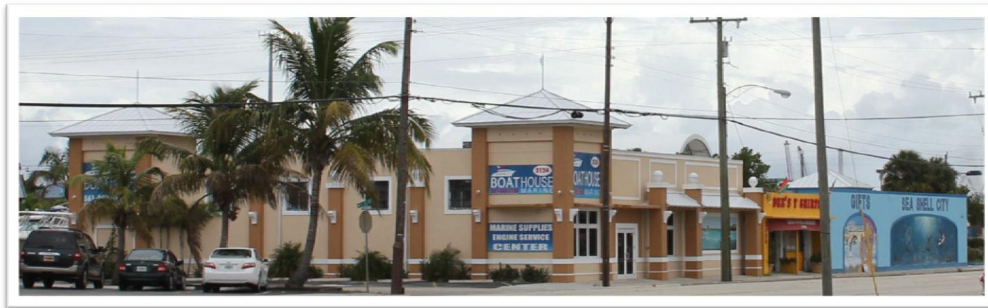
Figure 12 Boathouse Marine After Receiving the Facade Improvement Grant
