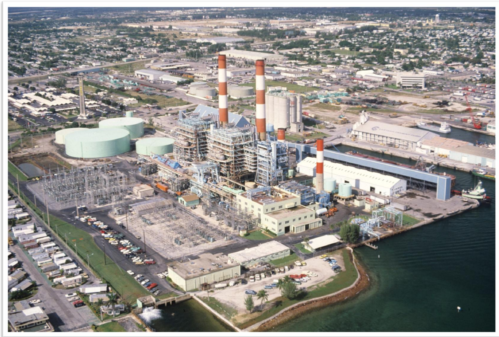
Figure 1 Outdated Inefficient Riviera Beach Power Plant
