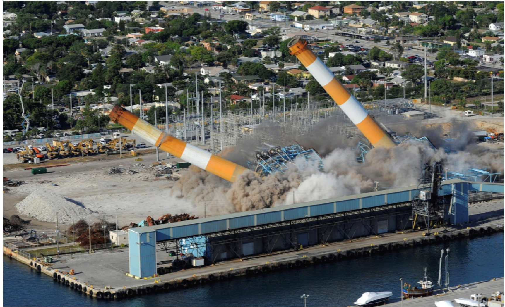
Figure 2 Demolition of Outdated Inefficient Riviera Beach Power Plant
